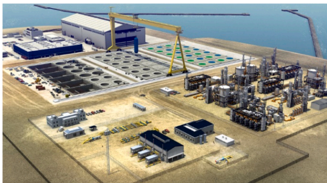
Fig. 11. Hydrogen Gigafactory with Factory in Back, Reactor Field in the Middle and Hydrogen Plant in the Front (Courtesy of LucidCatalyst (2020) ).
